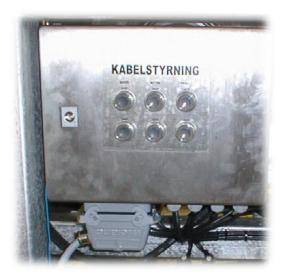
The adjustable controls for cable control is maneuvered from the buttons on the cable unit.
